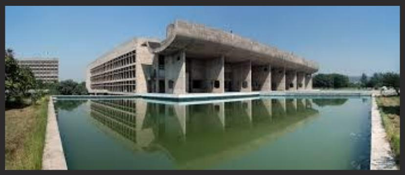
The utopian city of Chandigarh was designed by architect Le Corbusier in post-independence India and is largely built of concrete. Herein, the Palace of Assembly is situated on a reflecting pool with a sweeping sculptural form at the entrance which contrasts with the building's linear concrete columns throughout.
